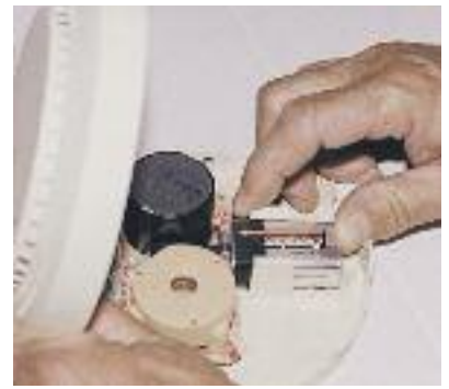
Replace the batteries for your smoke alarms every fall or when the alarm "chirps" and then test the alarms every month.
