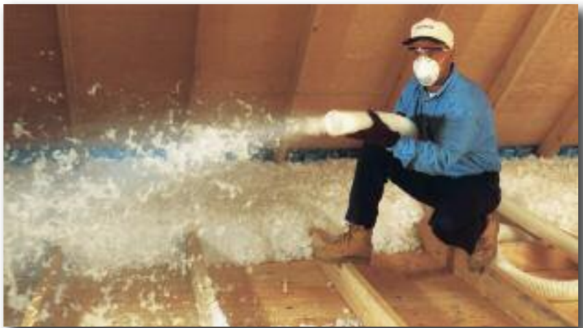
The effectiveness of insulation is measured in R-value per inch. The total R-value depends on the type and depth of the insulation.
