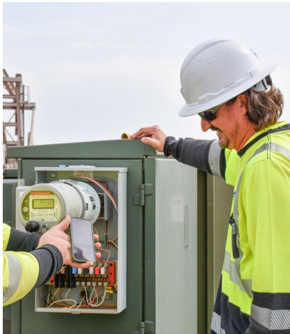
Journeyman lineworker Cody Braaten , checks meters.
