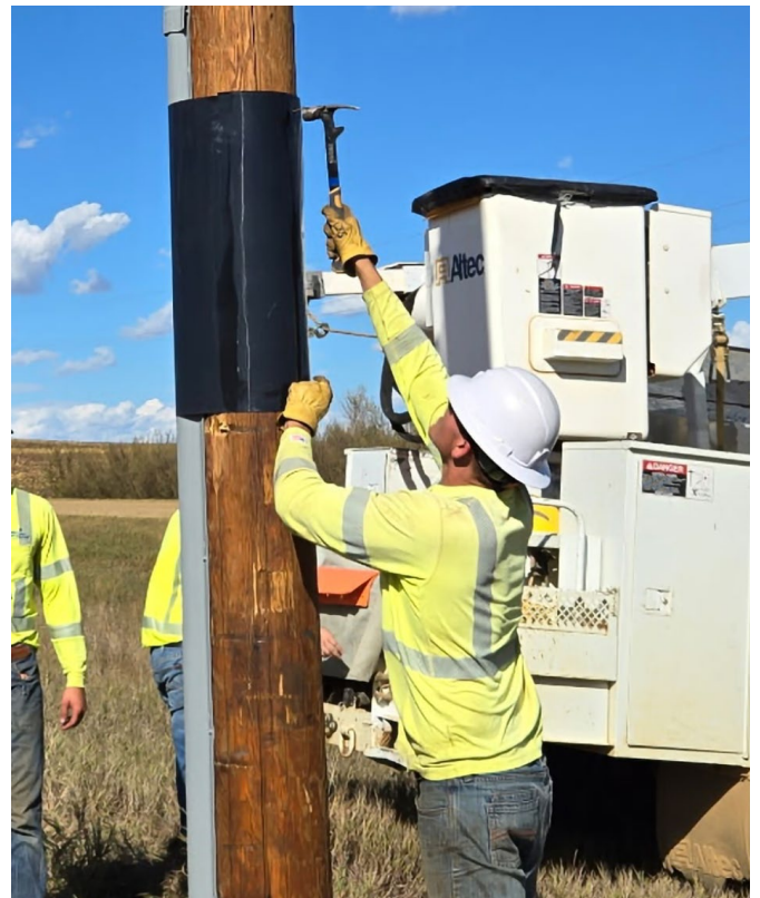
Line crews install ReliaWrap technology to poles.
